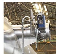
Bypass valve for EGB
