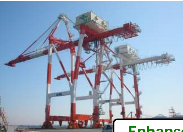
Energy saving PT
