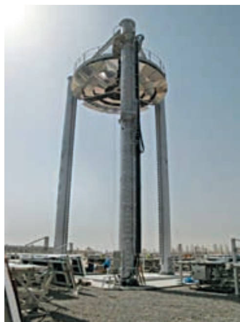
Center reflector tower and surrounding heliostats in experimental facility in Abu-Dhabi
