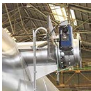
Bypass valve for EGB
