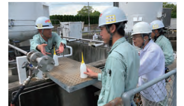
Renewal audit at the Oita Works
