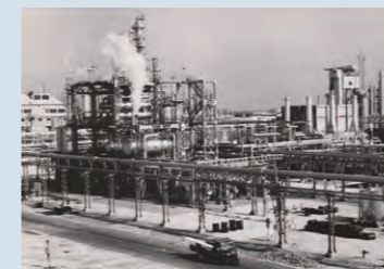
No.1 ethylene plant for Iwakuni Works of Mitsui Petrochemical Industries Ltd. (1958)
