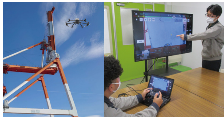
Using a drone to inspect a crane
