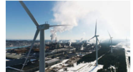
Mukaihama wind power plant
