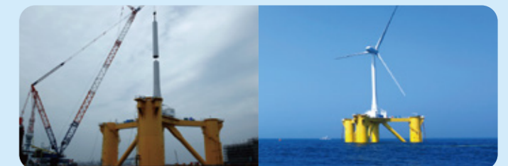
K Submersible floating wind turbine off the coast of Fukushima Fukushima Prefecture
