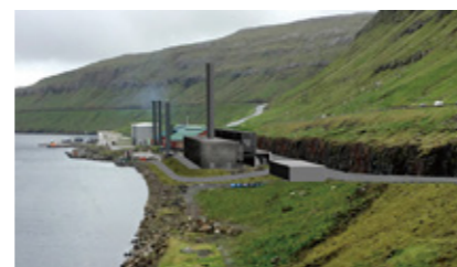
Diesel power plant for the Faroe Islands
