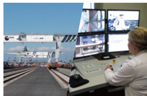
Container terminal automation system
