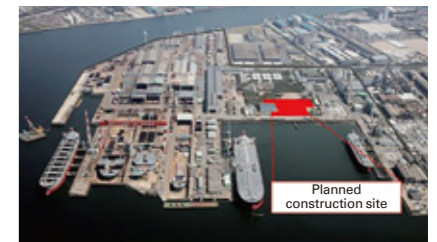
Planned construction site on the premises of Chiba Works
