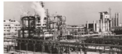
No.1 ethylene plant for Iwakuni Works of Mitsui Petrochemical Industries Ltd. (1958)
