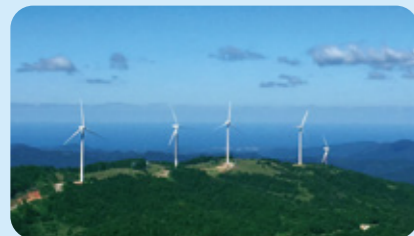
E Wind Farm Hamada Shimane Prefecture
