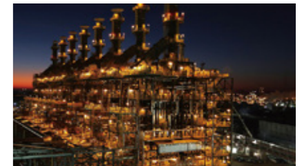
The completed cracker for the ethylene plant
