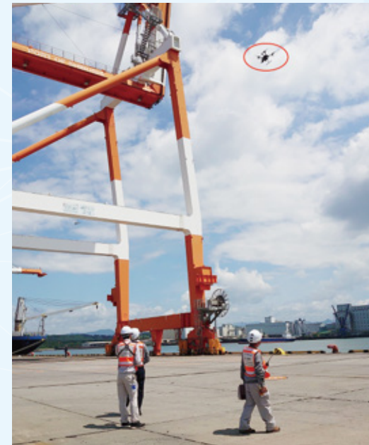
An inspection using an aerial drone
