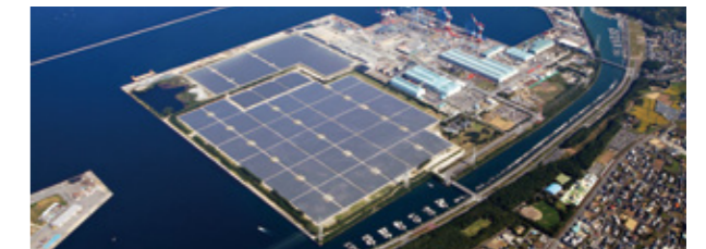
Panoramic view of the Oita Hiyoshibaru Mega-Solar Power Plant
