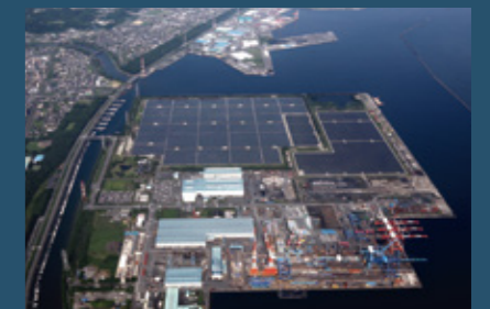
Ongoing improvement of the production capacity at Oita Works
