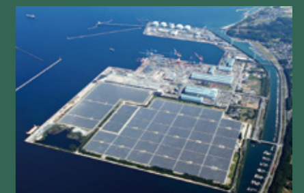
Full view of the Oita Hiyoshibaru Mega-Solar Power Plant
