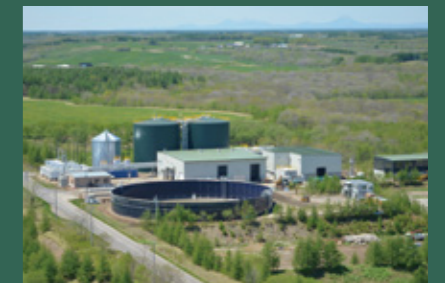
Betsukai Biogas Power Generation Plant
