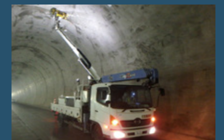
Investigation of tunnel lining concrete
