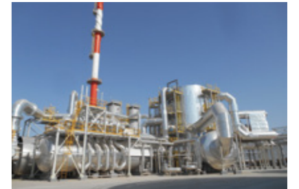
Sulfuric acid plant for Turkmenistan
