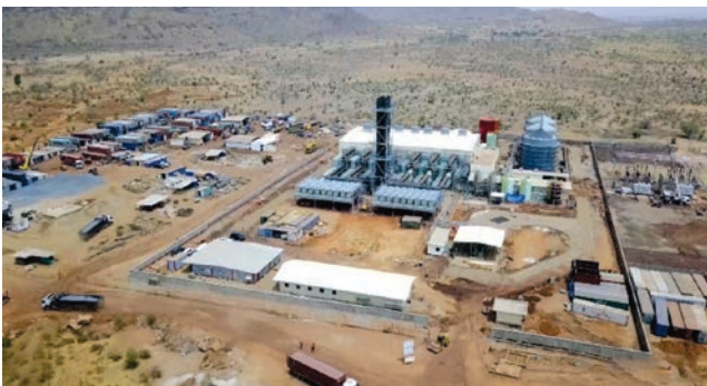
Photo 3 Mali Power Plant The 90 MW power plant recently inaugurated in Mali increases the country's power capacity by about 25 percent.
