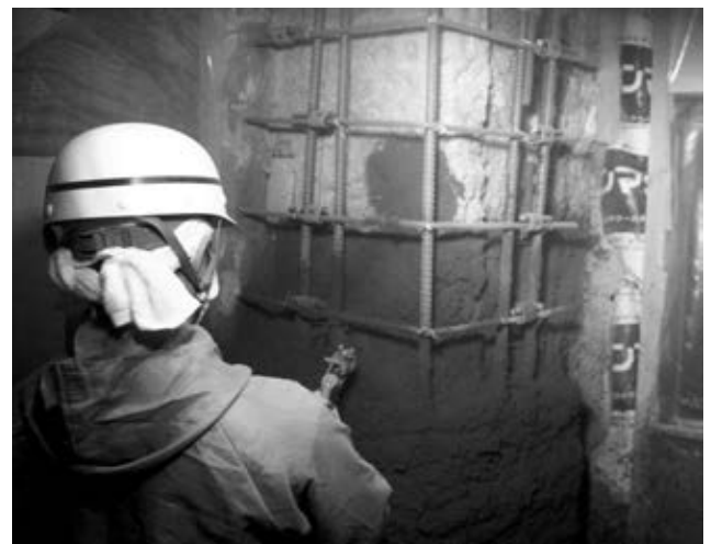
写真2 “なおしタル”施工状況 View of Spraying with NAOSHITARU
