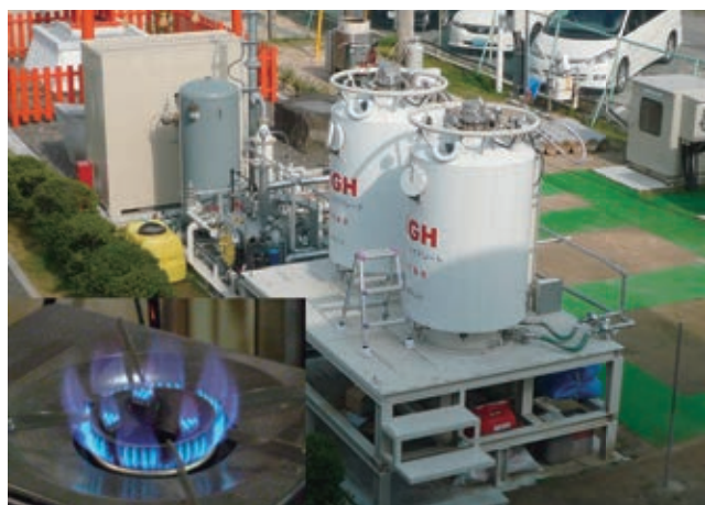
写真4 小口需要家ガス供給システムとコンロの燃焼状態 NGH Re-gasification System for City Gas and Combustion State at House Burner
