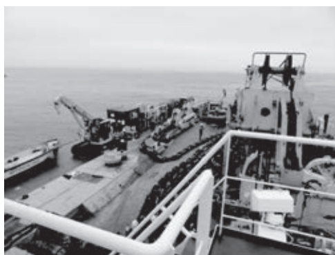
写真6 把駐力試験 Mooring Tensioning Test on the Barge
