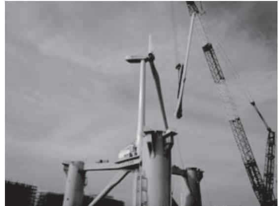
写真4 風車組立て状況 Assembling of Wind Turbine on the Floater
