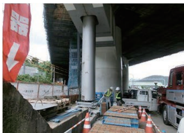
写真8 新設橋脚完成 New Bridge Piers Completed
