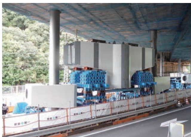
写真5 鋼製梁横取り・縦取り Longitudinal and Transverse Moving of Steel Beam
